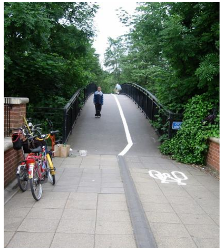
Queens Park Bridge over Markham Rd
