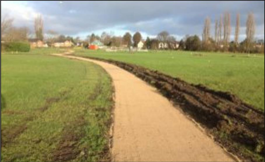
The Friends wanted to resurface the existing path surface and also build a new section across to Brampton Manor too. This meant that, unfortunately, asphalt would be too expensive and the money would only stretch to a 2 metre wide crushed stone surface plus drainage work to direct surface water under the path in the worst parts.
