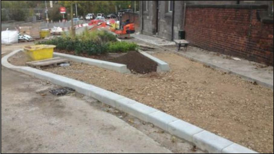
The work is being carried out by landscape architects TEP in partnership with Chesterfield Borough Council and incorporates a ‘rain garden’ which operates by diverting drainage from the road into a planted filter bed instead of going direct into the sewers.
