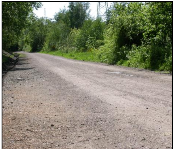
Widened track on the Trans Pennine Trail
